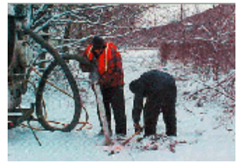
Figure #1. Field Crews completing test holes during winter conditions.
